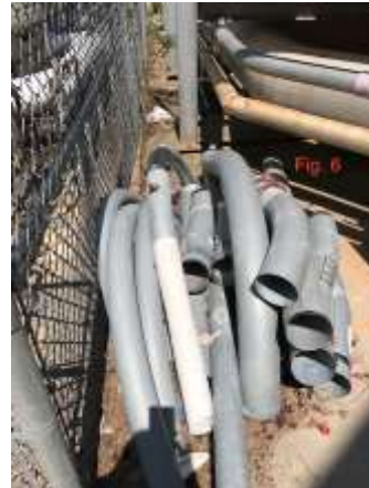
Figures 5, 6 and 7. NFPA 50 states the liquid oxygen 'farm' should be free of debris and plant life that may represent a fire hazard. Note the excessive amount of greenery and miscellaneous rubbish stored in and nearby the farm.
