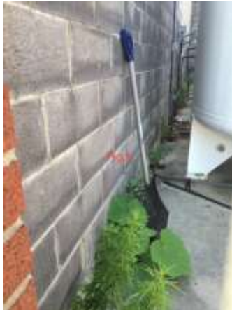
Figures 5, 6 and 7. NFPA 50 states the liquid oxygen 'farm' should be free of debris and plant life that may represent a fire hazard. Note the excessive amount of greenery and miscellaneous rubbish stored in and nearby the farm.
