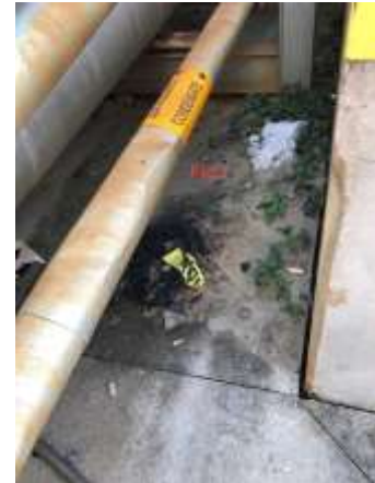
Figures 5, 6 and 7. NFPA 50 states the liquid oxygen 'farm' should be free of debris and plant life that may represent a fire hazard. Note the excessive amount of greenery and miscellaneous rubbish stored in and nearby the farm.
